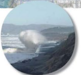
Taraval Seawall overtopping (1980s)
